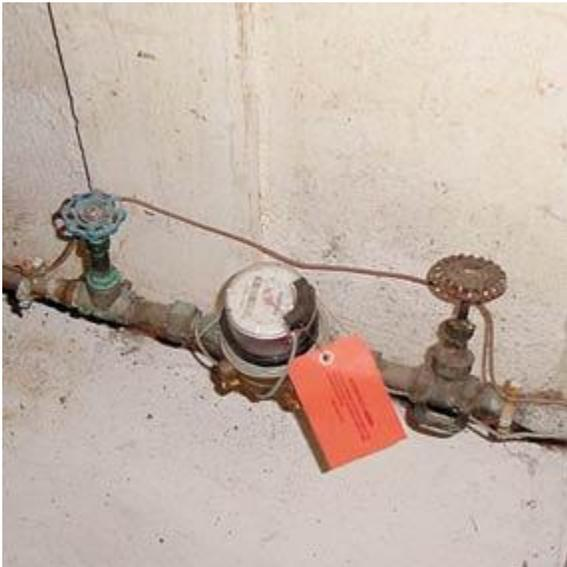
The valve on the right in this photo is the main shutoff; the valve on the left is the house-side main shutoff. In newer homes, these will probably be ball valves.
