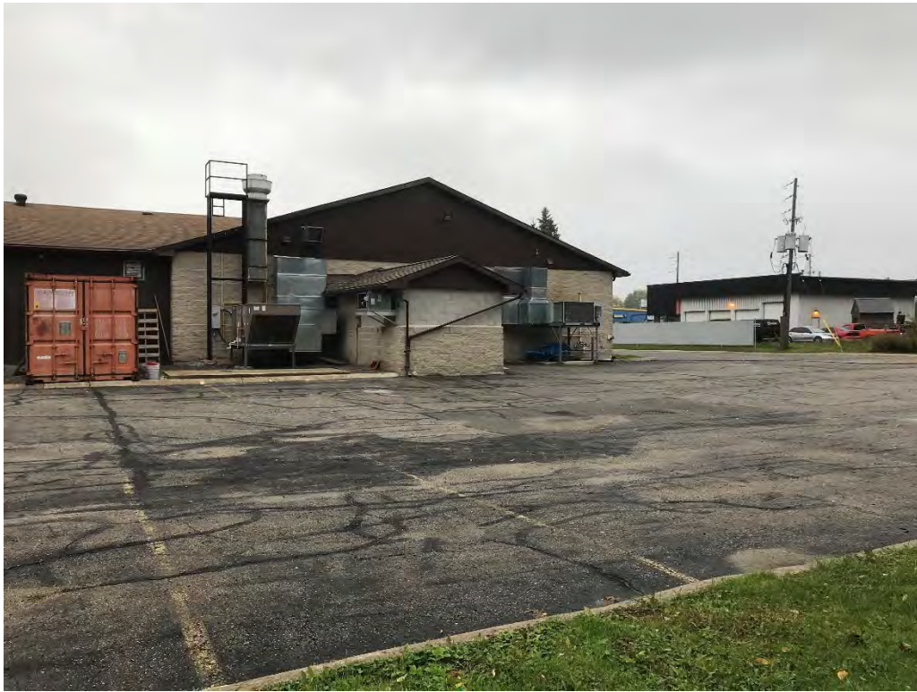
Photo 3: View of adjacent property to the west.
